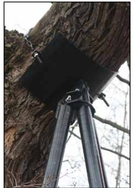
Top: The most likely scenario for this 200 year-old maple – the tree falls splits in half. Above: Cradle in situ on tripod support.
